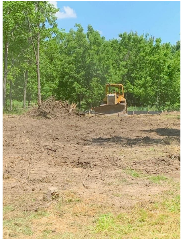
First day of construction at W.S. Gibbs Memorial Park - June 16, 2020.
