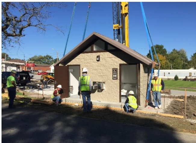
Installation of the restrooms at the Coatesville trailhead, 2018
