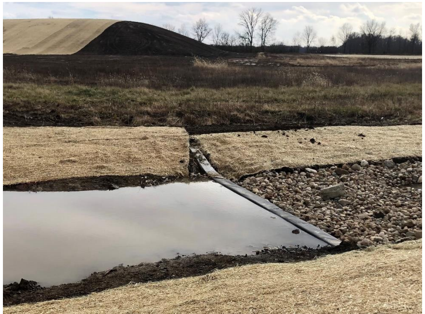
Forebay weir and erosion control / natural water filtration system at W.S. Gibbs Memorial Park. Turf grass blankets can be seen on the hill in the background. Prairie grass blankets were added on the ends of the hill after this photo was taken.
