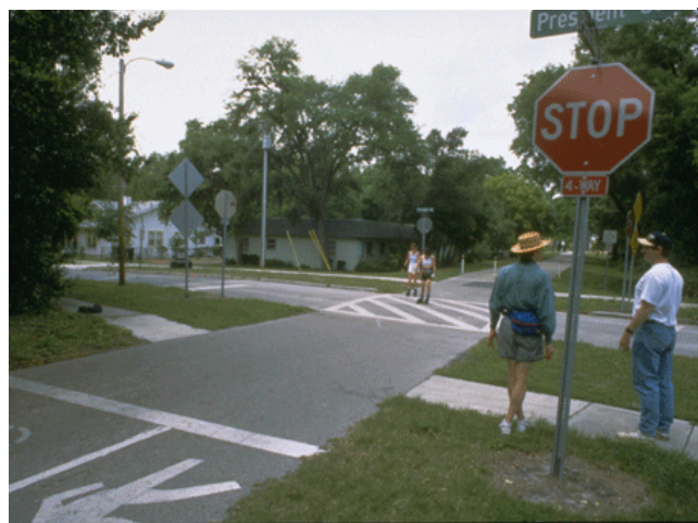
Road crossing, with signage for both vehicles and trail users. Photo courtesy of Daniel Burden.
