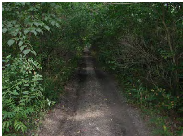
View looking east from the existing bridge showing overgrown conditions along top of the elevated former railroad corridor. Source: Storrow Kinsella Associates Inc
