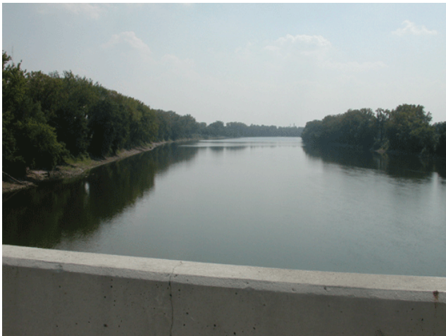
View of the Wabash River looking south from the eastbound U. S. 40/National Road bridge sidewalk. Source: Storrow Kinsella Associates Inc
