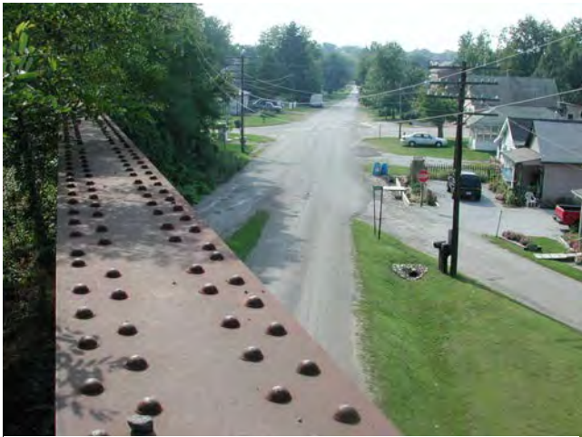
View looking from the elevated bridge out over the Historic National Road below. Source: Storrow Kinsella Associates Inc
