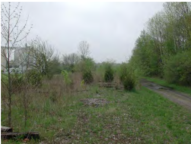
View showing unearthened railroad ties along the corridor near the C. R. 150 W crossing. Source: Storrow Kinsella Associates Inc
