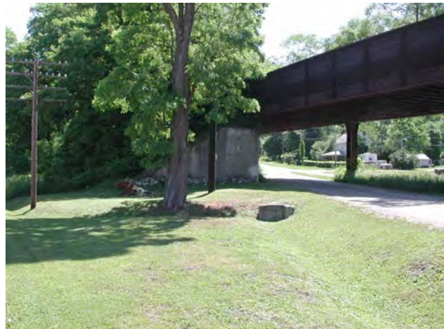
View of the existing elevated corridor, railroad bridge, and possible site where a trailhead may be developed. Source: Storrow Kinsella Associates Inc
