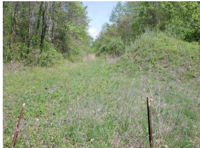
View of the elevated corridor, which leads down to C. R. 675 W. Source: Storrow Kinsella Associates Inc
