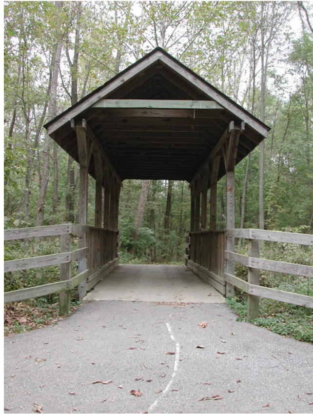
This is an example of a newly constructed bridge for a trail crossing a stream. Photo courtesy of Storrow Kinsella Associates Inc.
