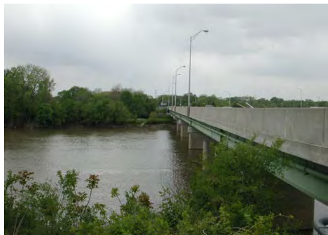
The U. S. 40/National Road bridge spans the Wabash River west of Terre Haute. Source: Storrow Kinsella Associates Inc
