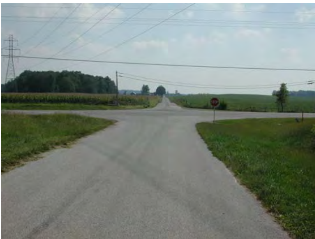
View looking south along Swallow Road toward the U. S. 40 intersection. Source: Storrow Kinsella Associates Inc
