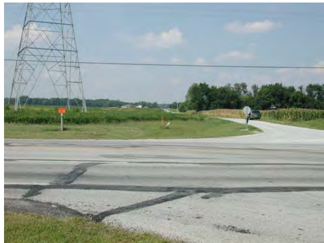
View looking north from the U. S. 40/Swallow Road intersection. Source: Storrow Kinsella Associates Inc
