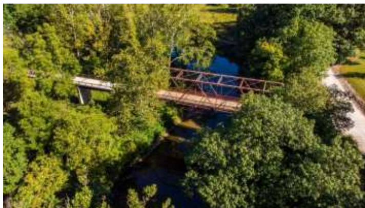
Aerial View of McCloud Nature Park. Source: Dave Novak.
