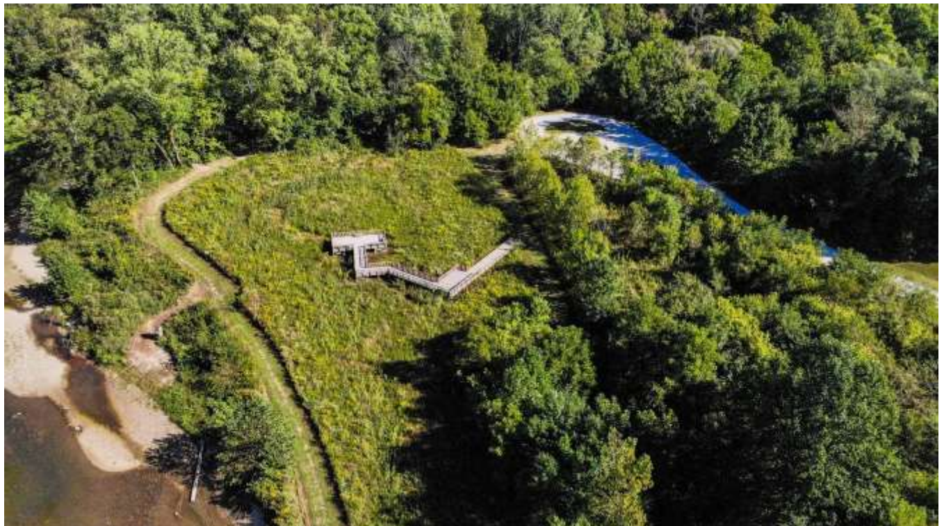
Aerial view of wetland habitat, boardwalk, and observation deck at McCloud Nature Park. Source: Dave Novak.
