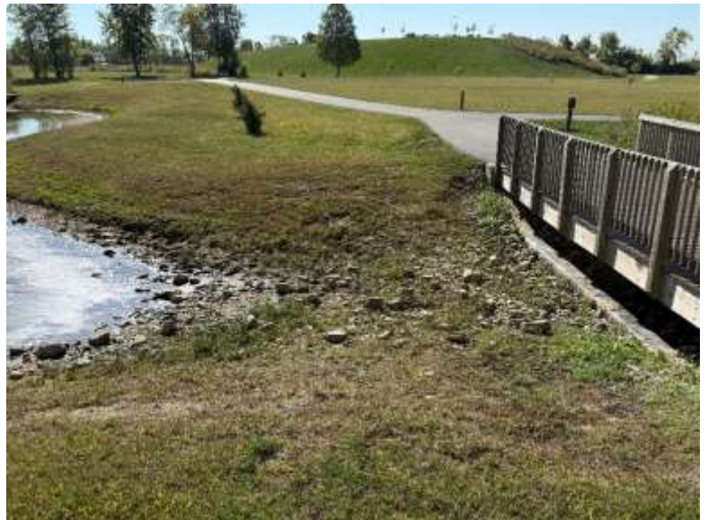
Forebay weir and erosion control / natural water filtration system at W.S. Gibbs Memorial Park.
