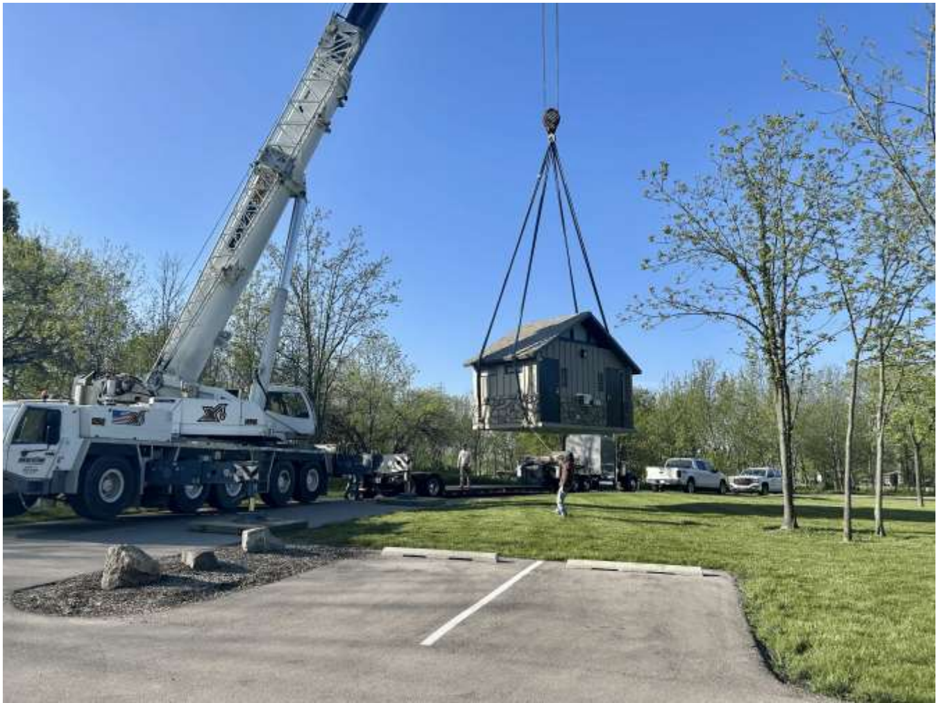
Installation of the CXT Denali restroom at W.S. Gibbs Memorial Park.
