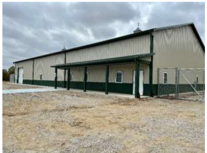
Exterior of the Gibbs maintenance hub after construction
